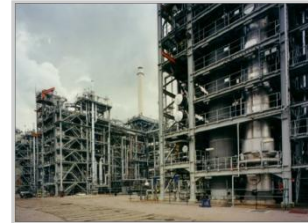
Shell Pernis 1997 Cracked Residue 3x550 t/d
